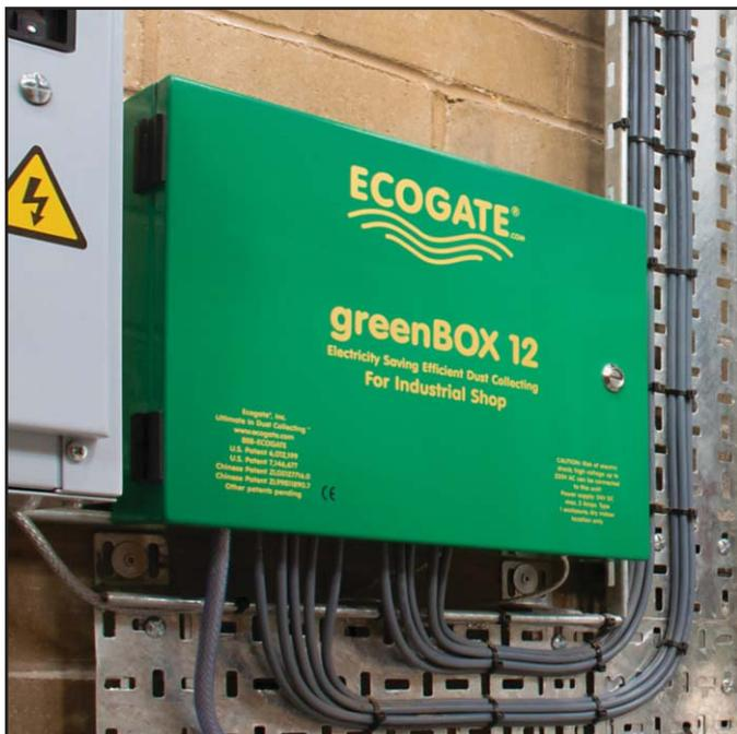
*Ecogate® greenBOX 12 controls the variable speed drive inverter unit which adjusts fan speed to match machine usage.*
