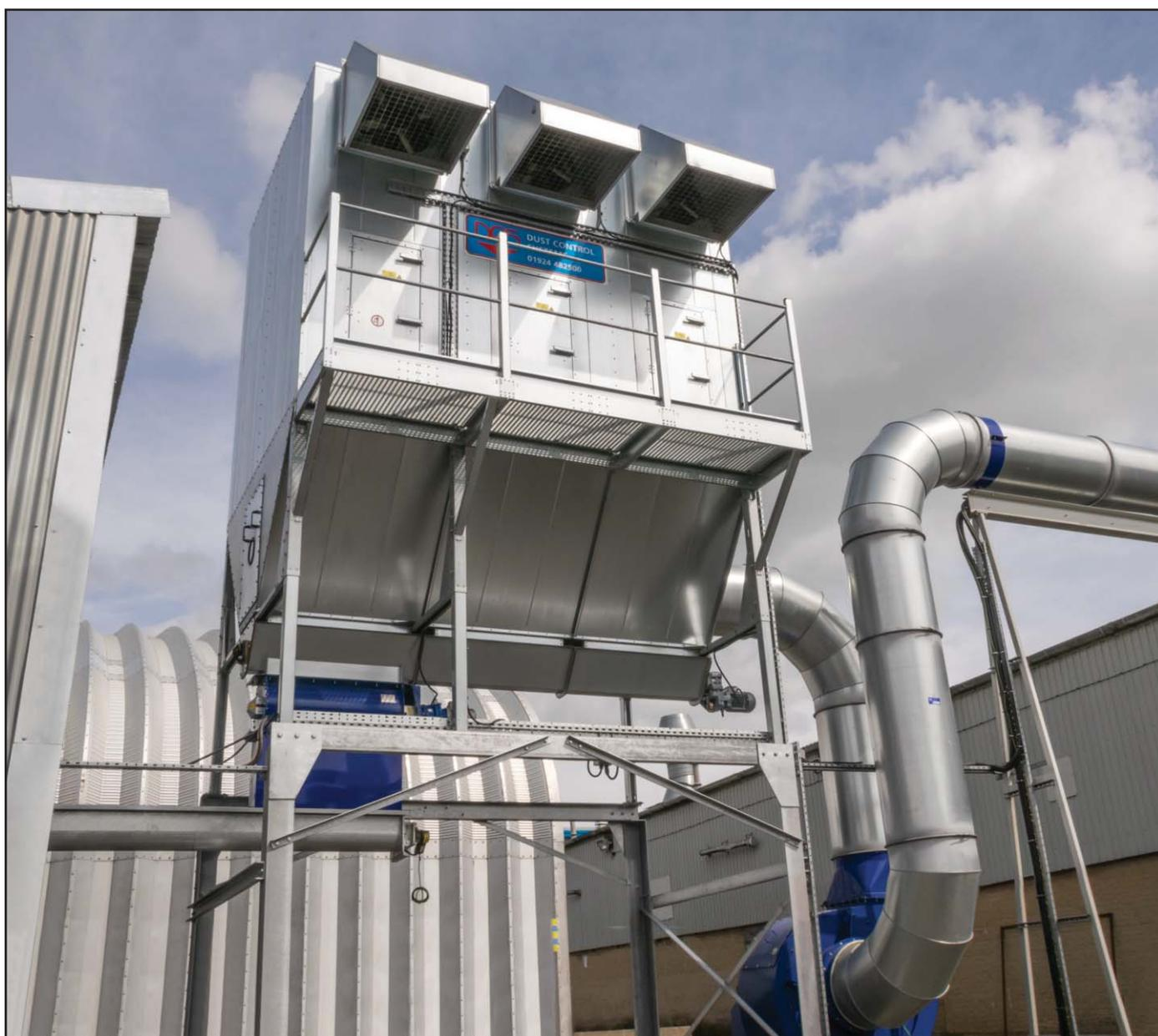
*DCS installed an NFSZ3000 3HJLR modular filter with 45 kW main fan and rotary valve.*
